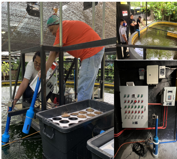
Automated Control and Monitoring System for Recirculating Aquaculture System (RAS)
